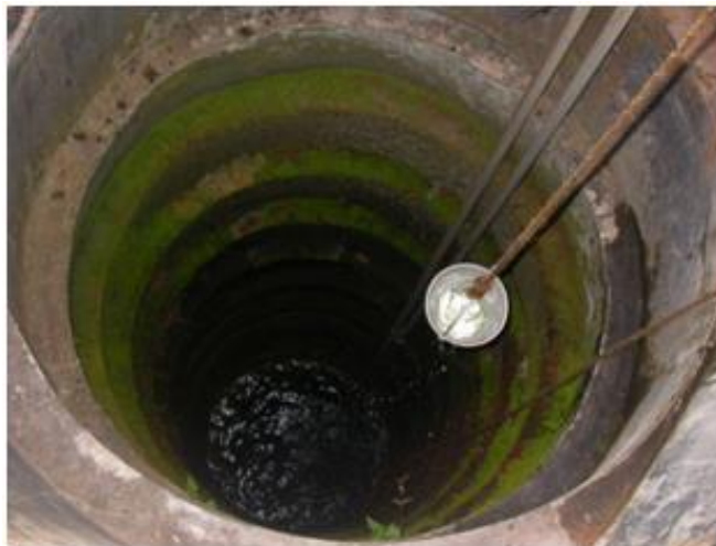
Fig 2.3 sample 3 location Well in NMAMIT
